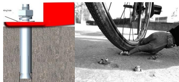
Figure 1.2 Difficult removal of expansion bolt
